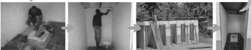
In the process of renovation / 修繕の様子
